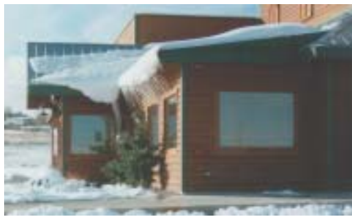
The icicles at center are about to break the front windows when this bank of snow slides farther.
