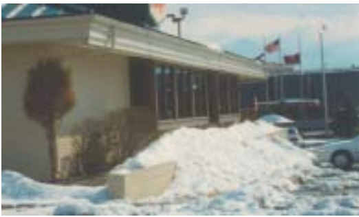
Fortunately no one was using the pedestrian walk at above left when this avalanche occurred.
