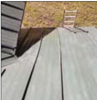
The snow retention system on this roof was not engineered for the snow loads. The sliding snow impacted the retention system, tearing it from the panel seams.
