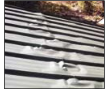
As the snow moved down slope in the valley area, the panel seams tried to force the snow to compact denser. Eventually the force of the snow put enough lateral pressure on the roof system to push the panels sideways. The panels buckled at mid slope, unseaming the panel at the end of the valley and...
