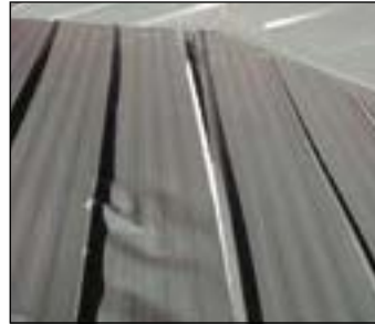
As the snow moved down slope in the valley area, the panel seams tried to force the snow to compact denser. Eventually the force of the snow put enough lateral pressure on the roof system to push the panels sideways. The panels buckled at mid slope, unseaming the panel at the end of the valley and...
