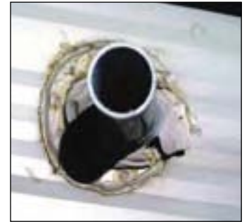
These pipes were left unprotected and have suffered damage due to sliding ice and snow.
