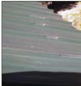
The snow retention system on this roof was not engineered for the snow loads. The sliding snow impacted the retention system, tearing it from the panel seams.
