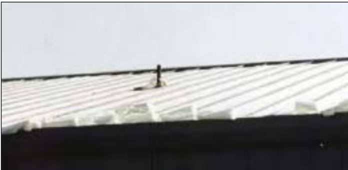
This picture shows how sliding snow reacts when encountering an obstacle such as a pipe penetration or gutter.
