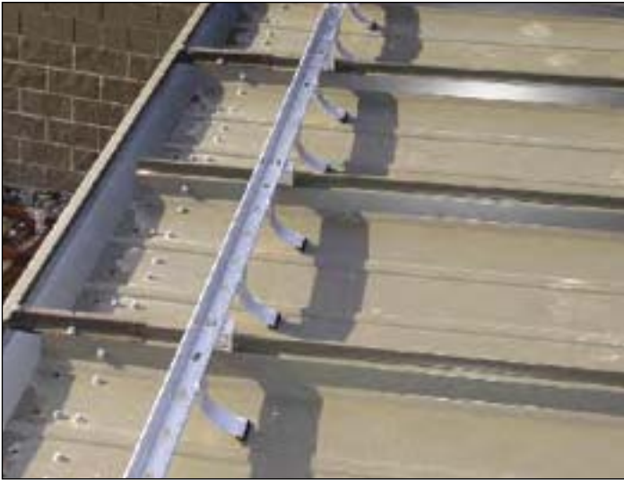
S-5! ColorGuard snow retention system installed at the building eave utilizes clamps that attach to the panel seam without penetrating it.
