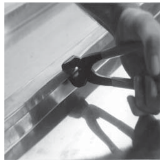
Finishing batten seam at a clamp location
