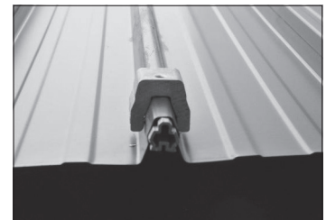
Example of correctly installed S-5-KHD clamp
