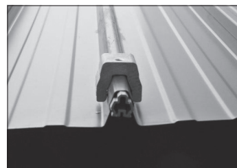
Example of correctly installed S-5-KHD clamp
