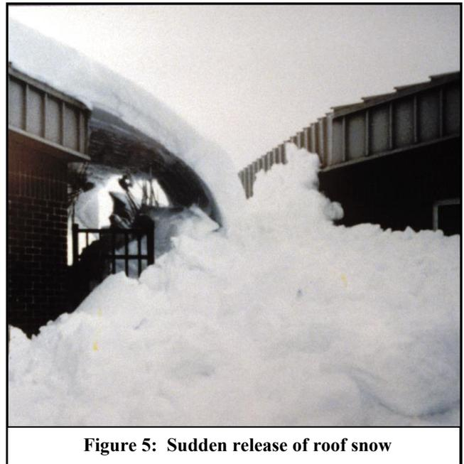
**Figure 5: Sudden release of roof snow**
